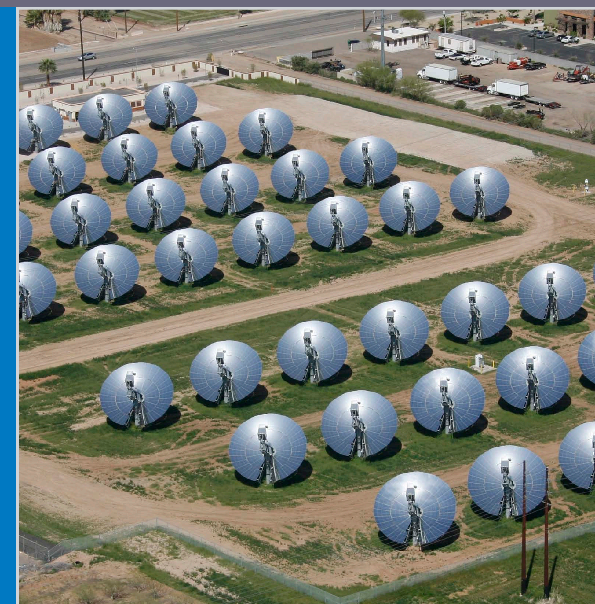
Each parabolic dish uses a Stirling engine to generate 20 kW of power at Maricopa Solar Power Plant in Arizona.
