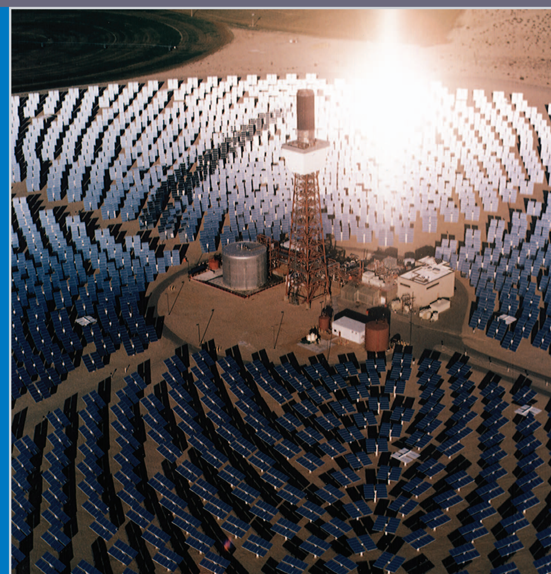
This 10-MW power tower facility known as Solar Two near Barstow, California, demonstrated molten-salt storage.
