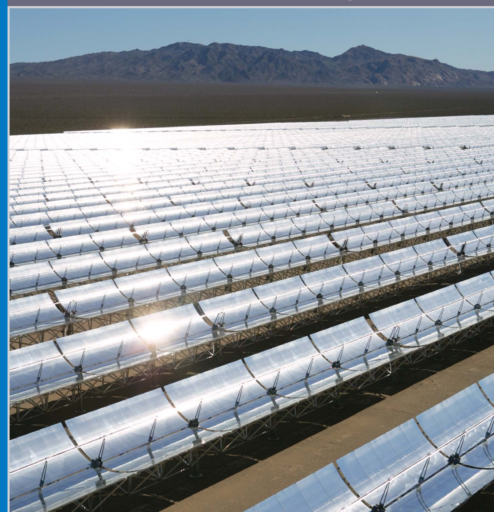
A section of the parabolic troughs from the Nevada Solar One project tracking the sun.
