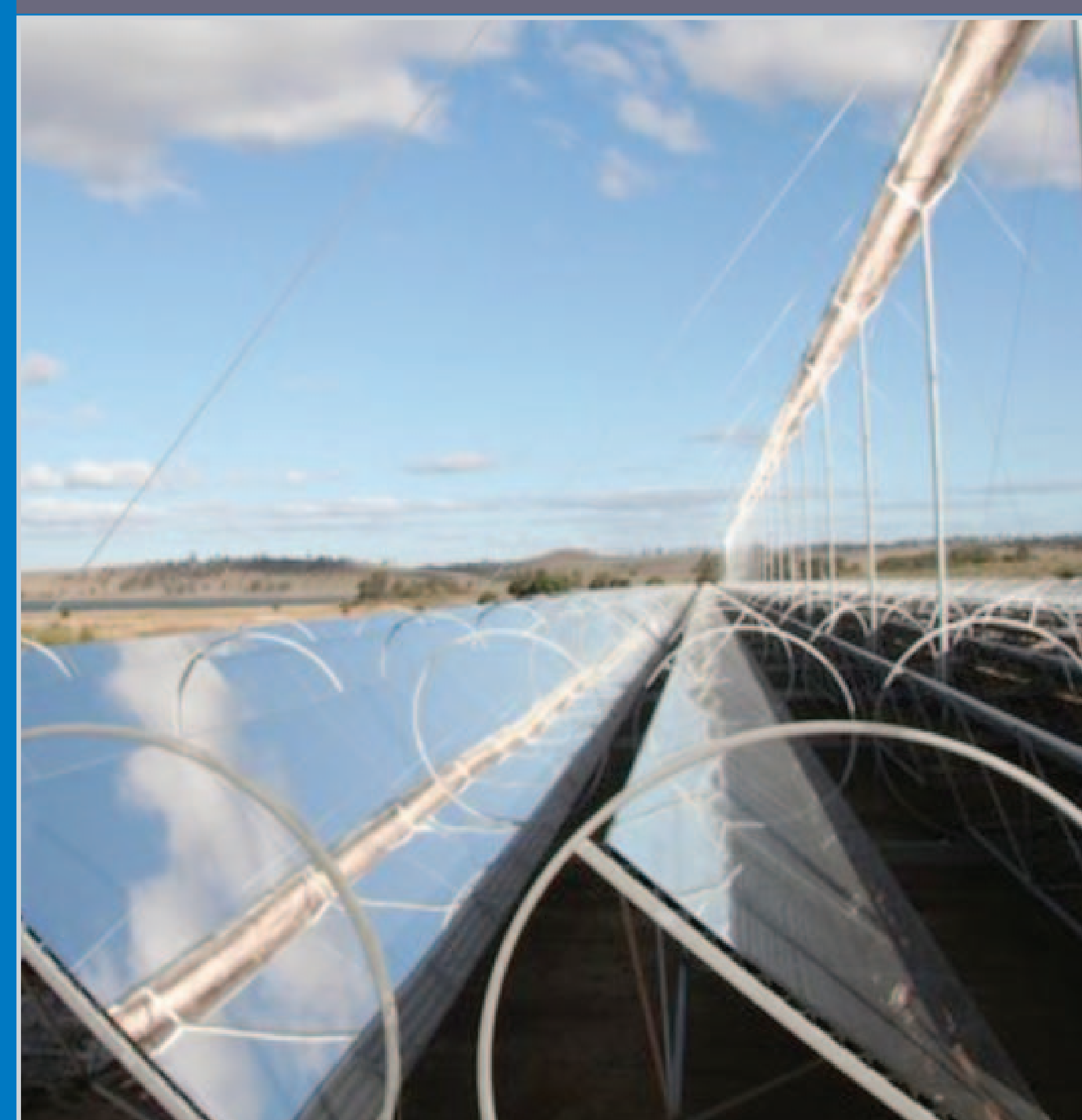
Close-up of linear Fresnel reflectors focusing sunlight onto a receiver.
